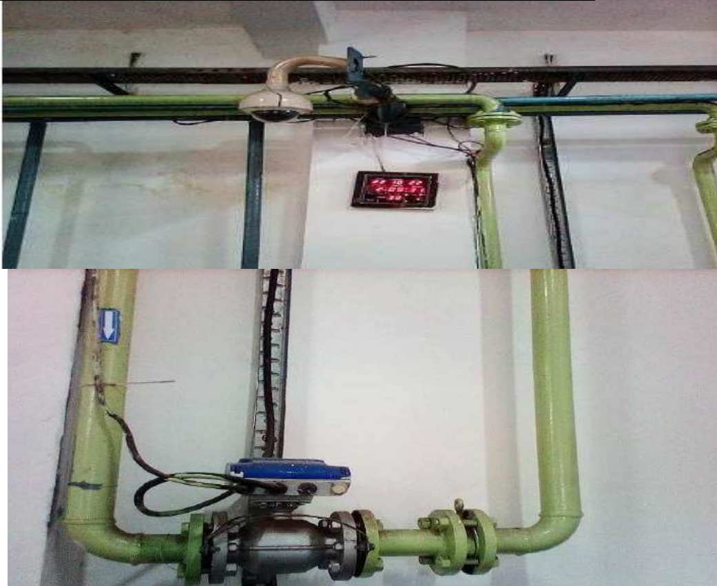
PTZ camera and digital flow meter
