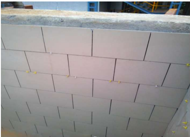
Impervious lining for Effluent tanks
