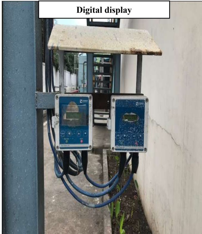
Flow meter and camera installation at ZLDS RO-Permeate outlet
