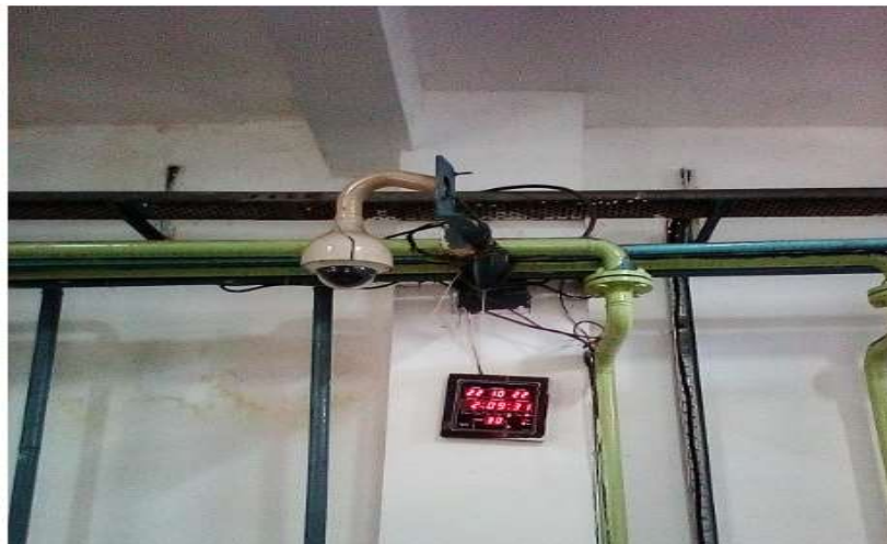
Flow meter and camera installation at ZLDS RO-Permeate outlet
